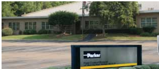
Fluid Control Division Facility, Madison, MS.
