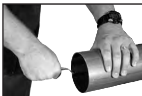
Figure 3: Deburr inside diameter deburring tool
