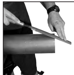
Figure 4: Deburr outside diameter using a half-round file
