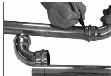
Figure 3 — Inserting the tube to proper depth
