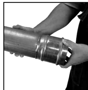
Figure 9: Inspection of final crimp
